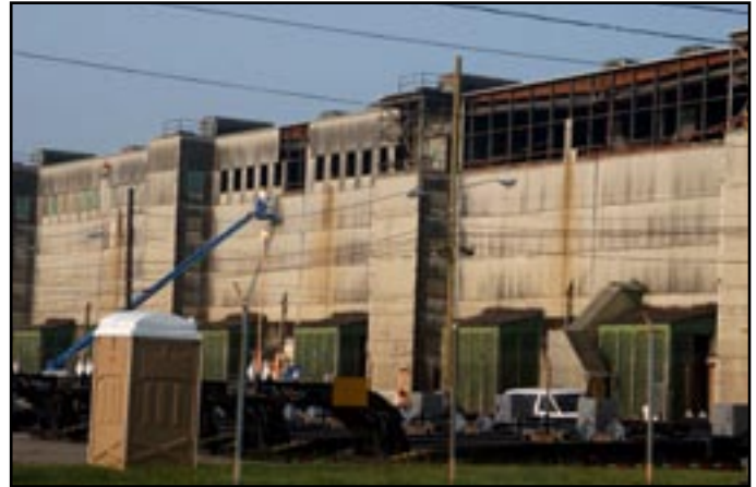
Removal of transite panels from the K-25 Building
