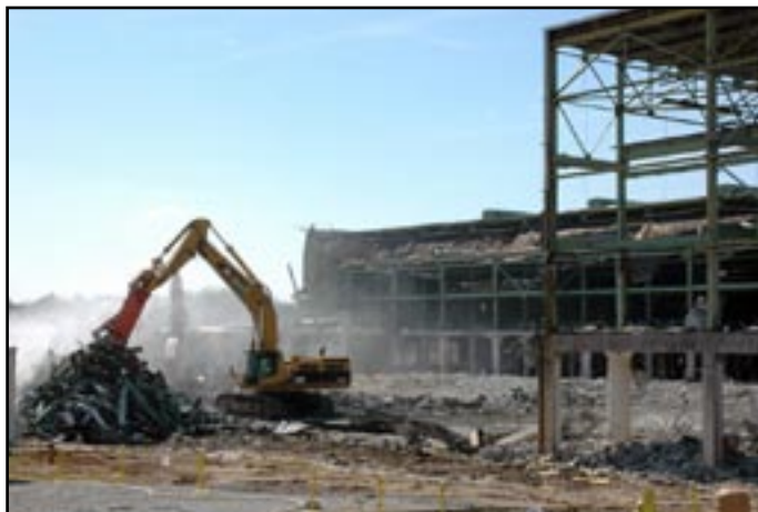
Demolition of K-29
